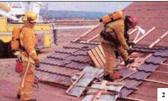
A "head" cut across and high on the roof makes it possible to peel back the metal roof panels (beginning at the top and working towards the bottom) with a rubbish hook.
