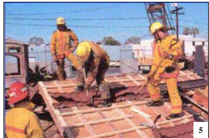
While being lightweight, the shape stamped into the metal makes the panels strong. They can easily be cut with an axe or carbide-tipped chain or circular saw. Though an axe is more than adequate, carbide-tipped chain saws cut through the metal very fast and can remove the sheathing at the same time.
