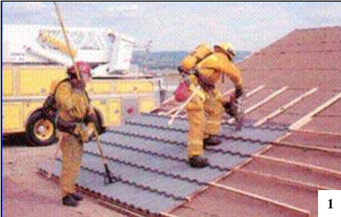
Firefighters investigate the roof assembly by cutting a small triangular inspection hole to reveal the substructure of the metal panel roof system. Photo 1 shows a 1 x 4 and 2 x 2 wood batten grid system nailed to the roof's framing.
