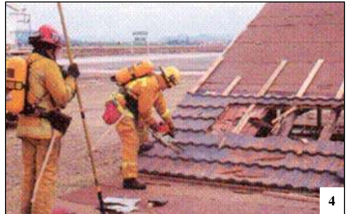
The metal roof may have been installed over an old existing roof such as; wood shakes or shingles, asphalt shingles, etc. The weight of the metal roof system would be less than 1.5 pounds per square foot.
