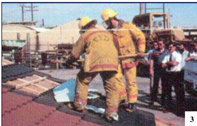
A pick-headed axe can easily lift the front of the panels away from the fasteners. Rubbish hooks are used to peel the panels away from the roof.
